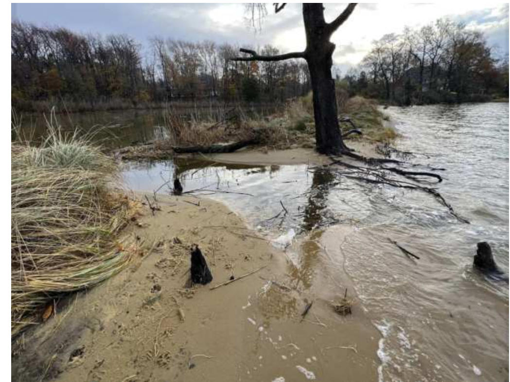
12/18 - Breach location with water flowing to the Chesapeake Bay / South River
