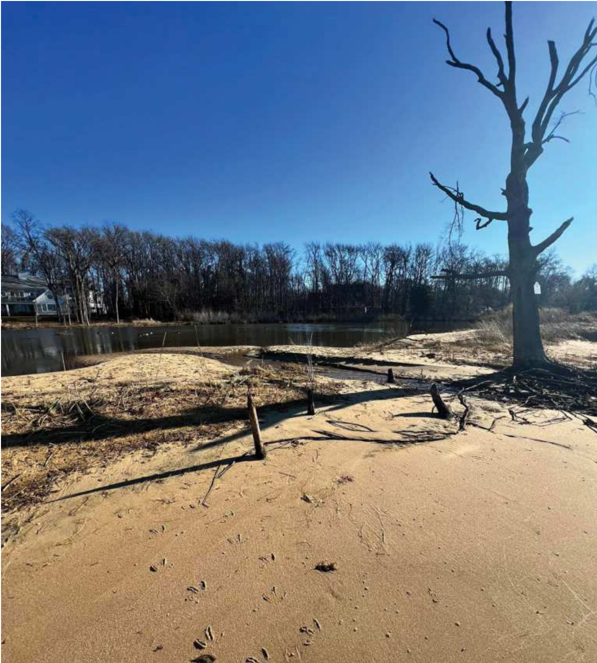
Berm Breach the day after the storm
